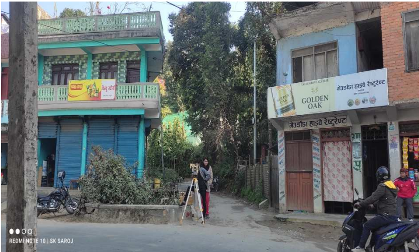
Bindu Shrestha House at start Chainage (L/S) before demolishing
