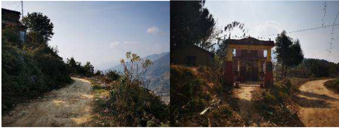
Existing road condition
