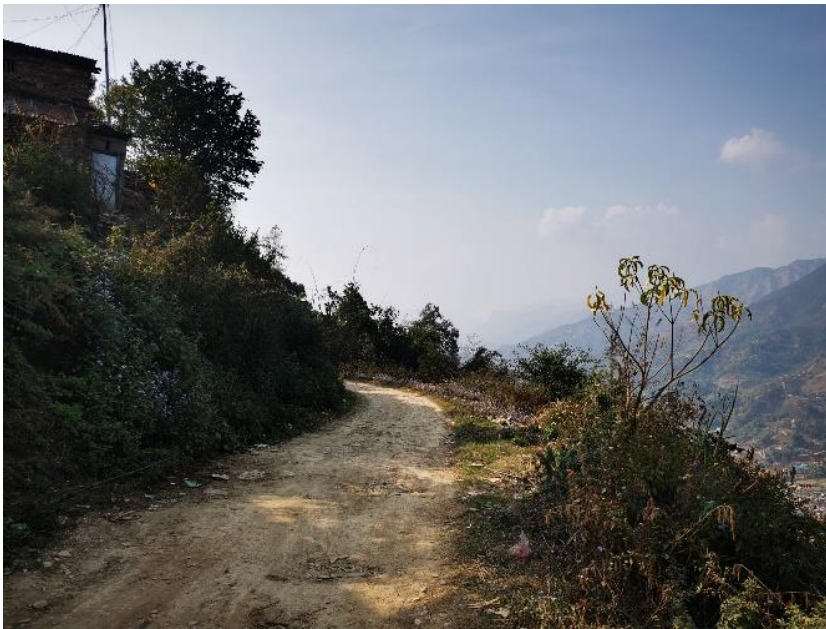
Existing road condition
