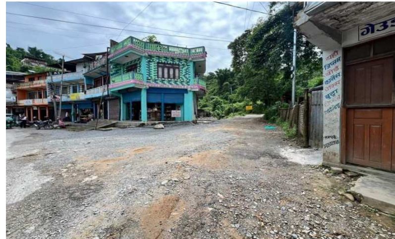
Bindu Shrestha House at start Chainage(L/S) after partial demolishing and reconstruction
